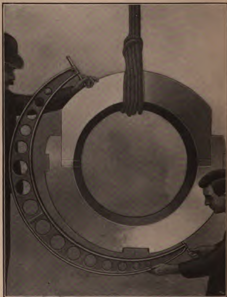
FIG. 221. — Large Micrometer.
